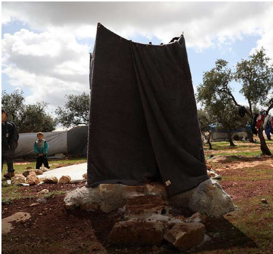
A toilet in an informal camp, a soak pit covered with canvas weighted down with rocks appears at the back where human waste is collected (source NoonPost)
