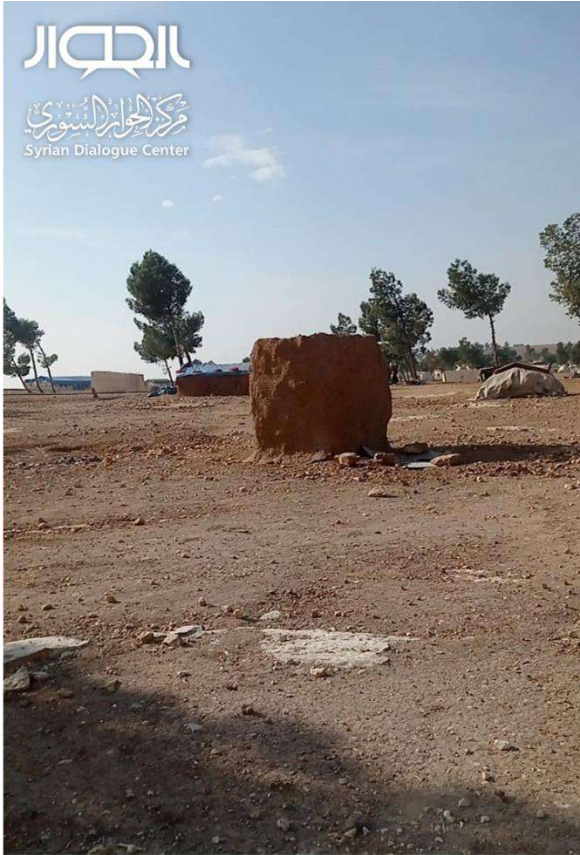
A toilet in an informal camp, made of a hole in the ground surrounded by three clay walls, one metre high, without any covering (private image)
